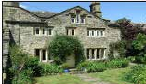
Grange Hall Cottages, Kildwick
